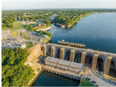
126MW Hydro, Pensacola Dam Grand Lake
