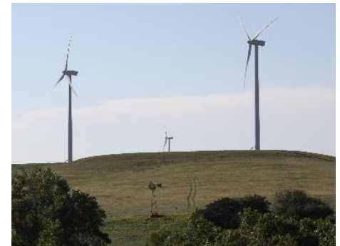
385MW Wind Across four projects
