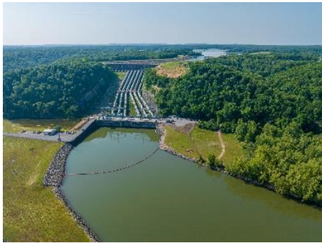
260MW Salina Pumped Storage Project W.R. Holway Reservoir
