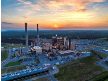
Combined cycle gas 495MW, Coal 492MW, Grand River Energy Center
