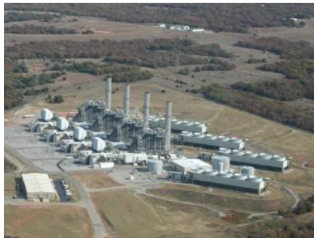
457MW Winter/435MW Summer Redbud Power Plant
