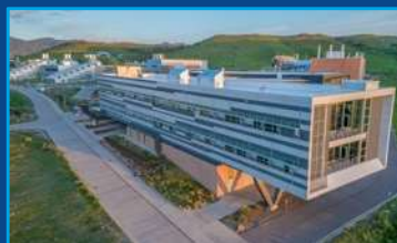
Energy Systems Integration Facility
